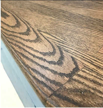
Laying the new flooring over the parquet, and from wing to wing turned out to be the most economical
